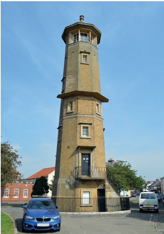
ABOVE: The high, rear light of a pair of leading lights established in the 17th century at Harwich. A low light was located on the beach some 200 m distant.
