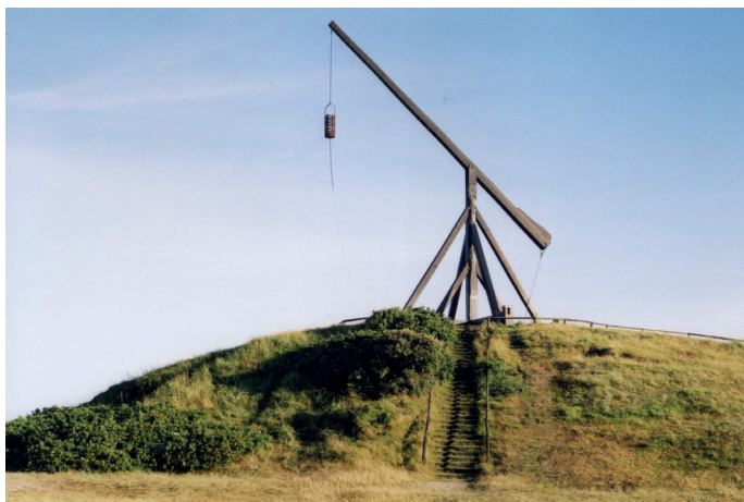
ABOVE: A replica of a swape light or vippefyr that was used at Spurn Head (1674). This one is at Skagen in Denmark, here on a hill rather than a stone tower.
