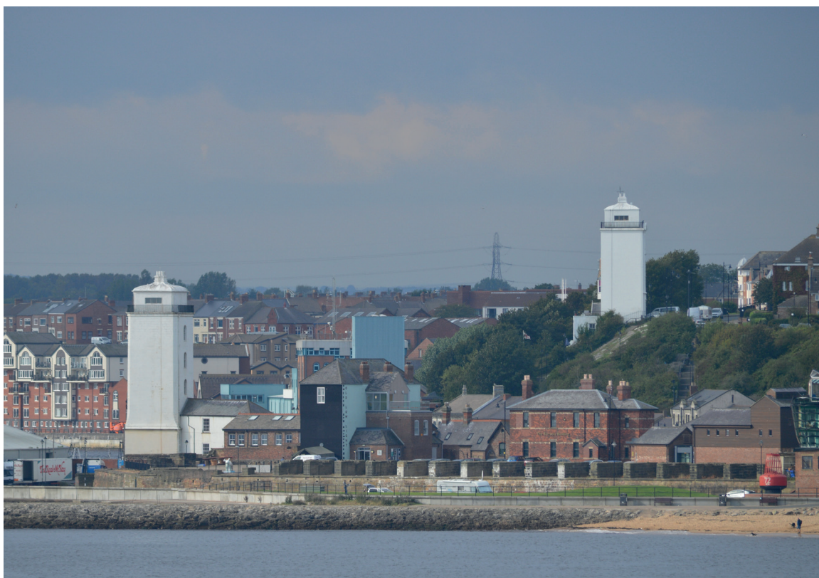
ABOVE: The two lighthouses at Tynemouth which, when aligned, show the safe channel into the River Tyne at Tynemouth. These two towers date from 1810 and replaced two earlier lighthouses of 1727, but the earliest lights were shown in similar fashion from 1540 after the granting of a Patent by Henry VIII to the Trinity House of Newcastle upon Tyne in 1536.
