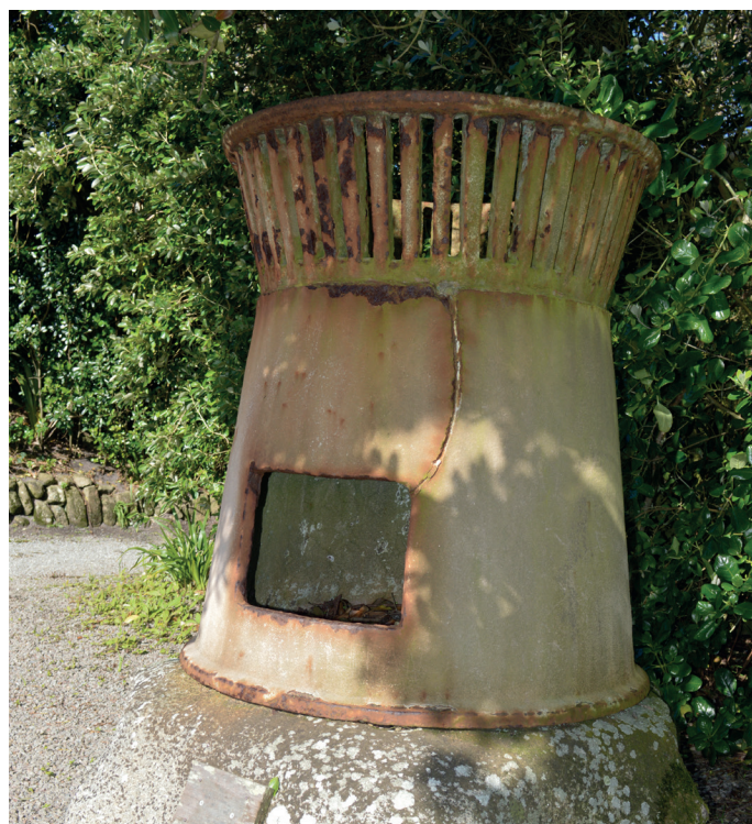
ABOVE LEFT: The St. Agnes lighthouse (1680) on the Isles of Scilly which was lit by coal burned in the cast iron chauffer (grate) ABOVE RIGHT. The unique item can be seen in the gardens of Tresco Abbey.
