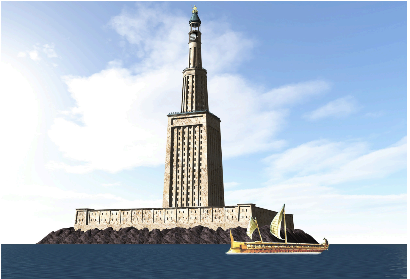
Fig. 5-14: An impression of the Pharos of Alexandria depicting the lighthouse surrounded by a 110 m square accommodation building, possibly constructed during the Roman period and used as a military barracks. It offered increased protection of the lighthouse from wave damage. The image offers the addition of a mirror mounted on the cylindrical section just below the lantern level. 124
